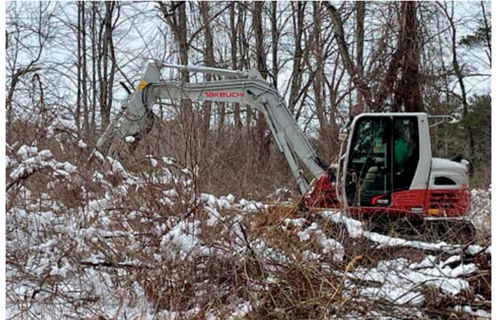
Mechanical clearing is the first step: removing dead trees and vines.
