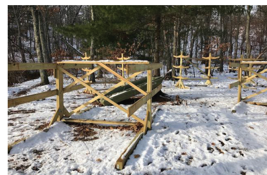
Storage racks like these will be used for canoes and kayaks
